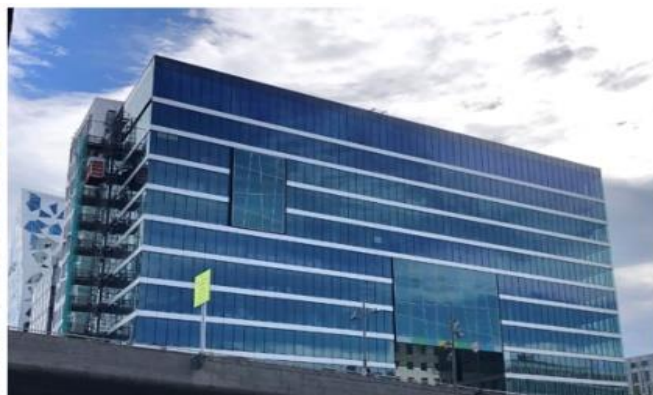
Highly insulative gas-filled multipane facade unit
