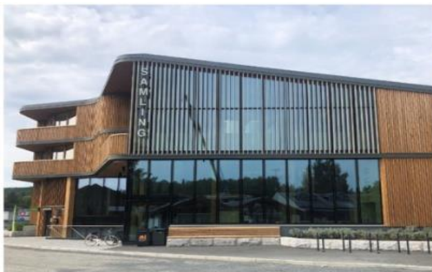
Highly insulative gas-filled multipane facade unit
